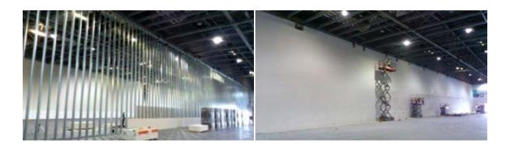
Deflection Head Details: Deflection head details are designed for each specific building taking into accoung roof crush factor and extreme wind loadings; please email <a href="technical@pjssolutions.co.uk">technical@pjssolutions.co.uk</a> we will be pleased to assist you.
